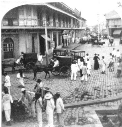
Rosario Street and Binondo Church from Pasig River, Manila, Philippines. Photo courtesy of the USAHEC.
