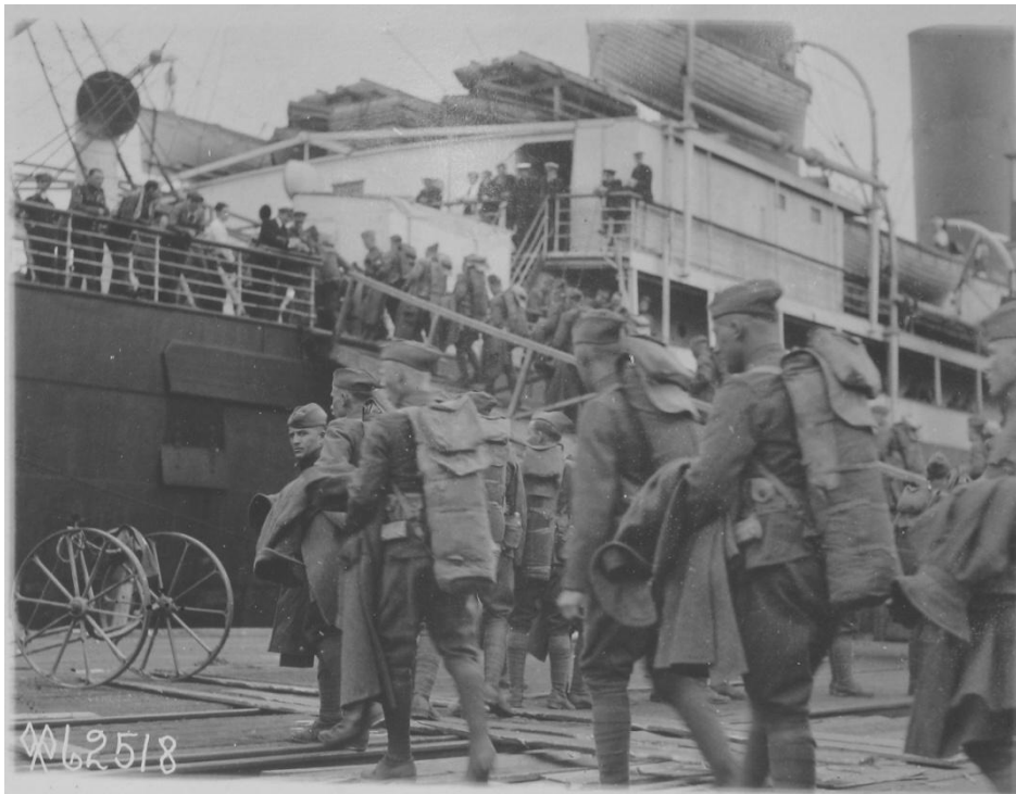
Co. L. 339th Infantry, embarking on the British transport "Czar" at Economia. This company was part of the first contingent to leave North Russia after wintering at Archangel. Economia, Russia. June 2, 1919. Photo courtesy of the USAHEC, World War I Signal Corps Collection.
